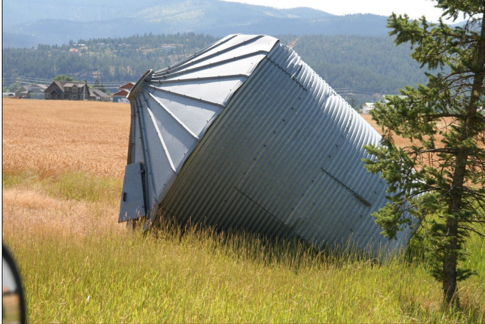
Figure 21 – Metal silo knocked over and damaged near Somers, MT (photo courtesy of Bryan Henry).
