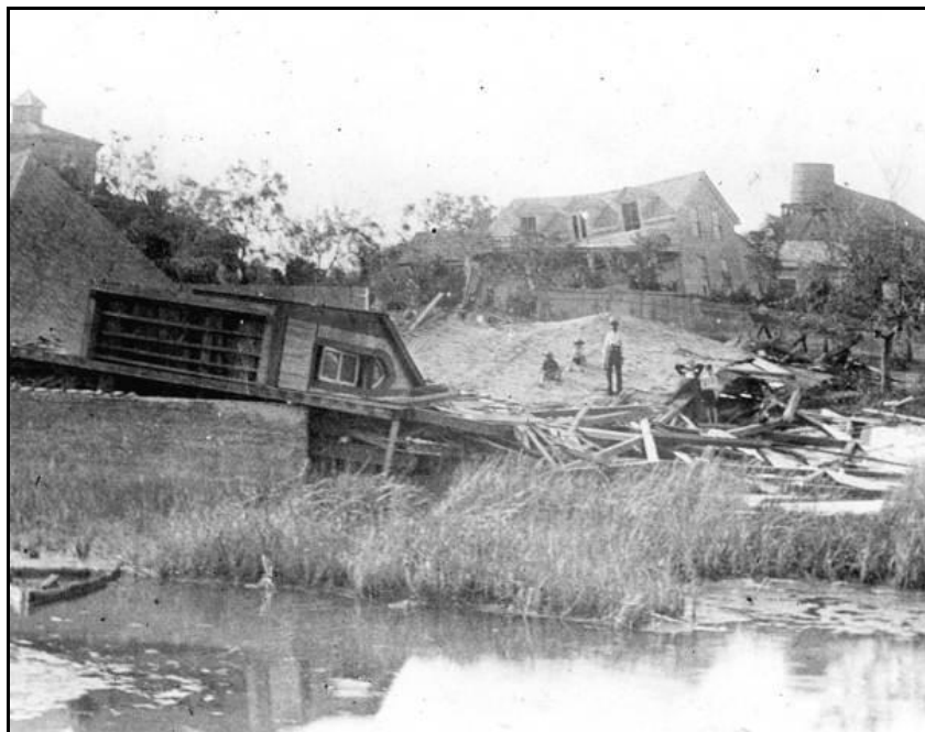
Figure 4. Damage to a house done by the powerful hurricane force winds, in Cedar Key, FL.
