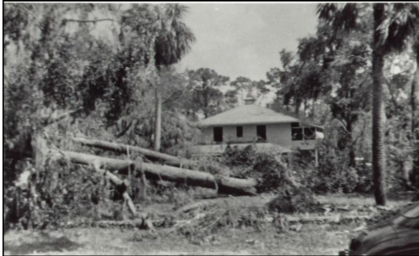
Figure 3. Fallen trees and other damage, in Yankeetown, FL.
