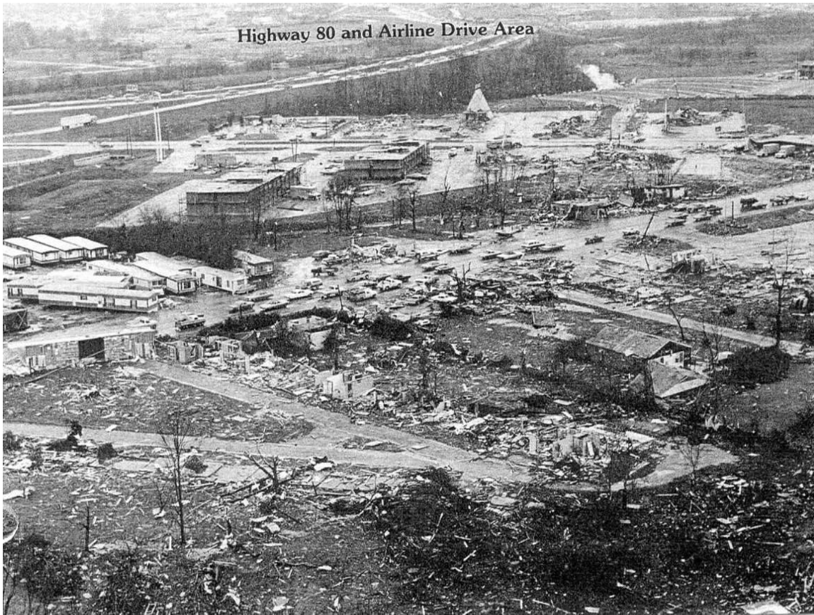
Figure 8. Damage at Hwy 80 and Airline Drive just north of I-20. Photo by Jack Barham. Reprinted with permission.
