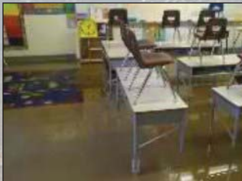
Flooded classroom at Saul Martinez Elementary due to a nearly stationary storm on September 11, 2012. (Source: KESQ TV)
