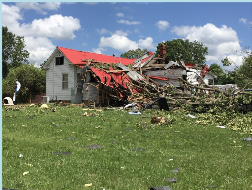
Damage from EF1 tornado in Eden, NC – May 5, 2017
