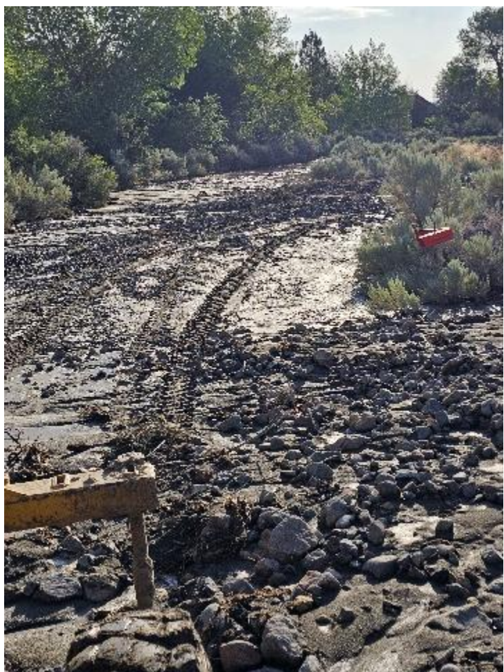
Photo 8: Flooding in Hoyo Canyon, Lyon County July 24th.
