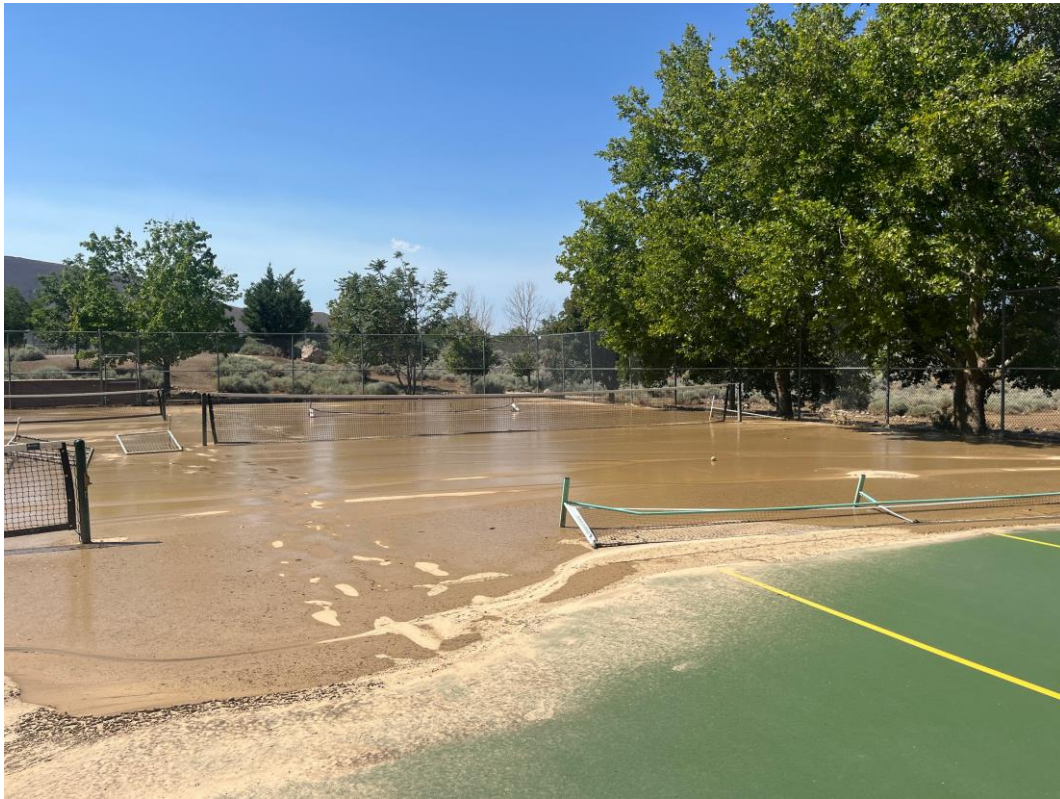
Photo 4: Tennis Courts in Hidden Valley Regional Park after July 21st flood event.
