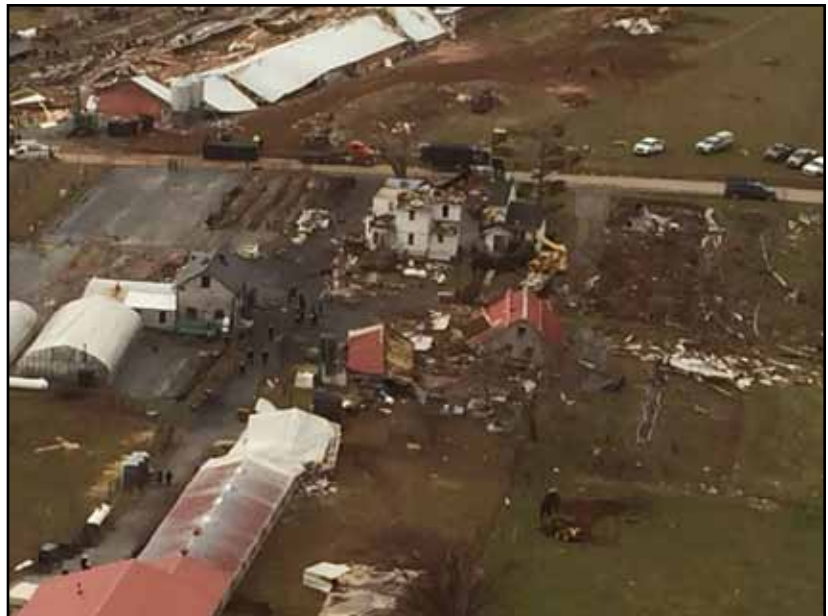
Damage caused by an EF2 tornado which struck near White Horse, PA, on February 24, 2016
