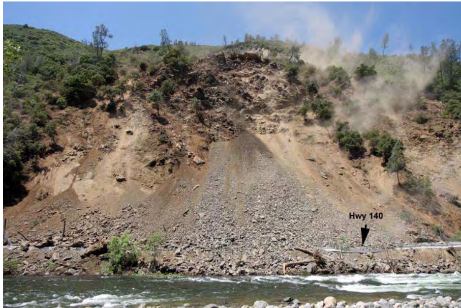
California State Highway 140 buried beneath a massive landslide on May 25th. Photo courtesy of Kome Ajise, CALTRANS District 10 Director, Stockton, CA.
