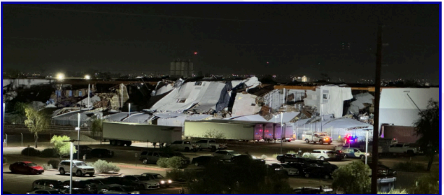
Complete collapse of warehouse roof near 47th Ave and Van Buren St. Photo by Cindy Kobold.
