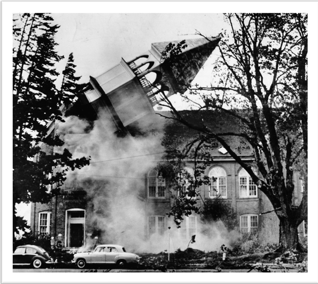
(above) Wind forces collapse of steeple on the historic Campbell Hall at the Oregon College of Education in Monmouth, Oregon on 12 October 1962.
