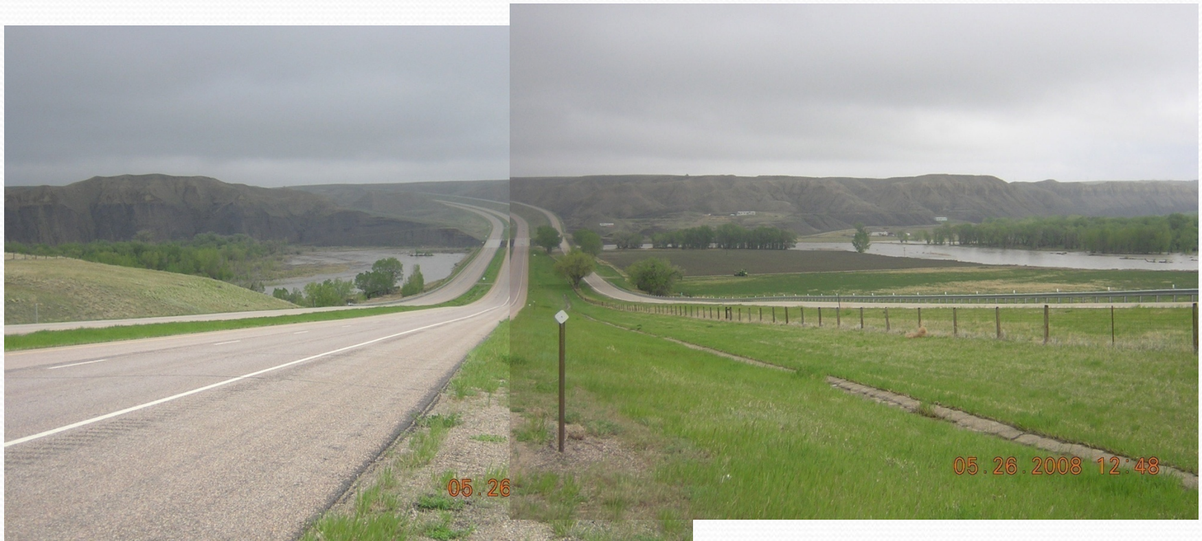
Shelby gage site ... looking north along I-15 05/26/2008 stage ~10.8 ft
