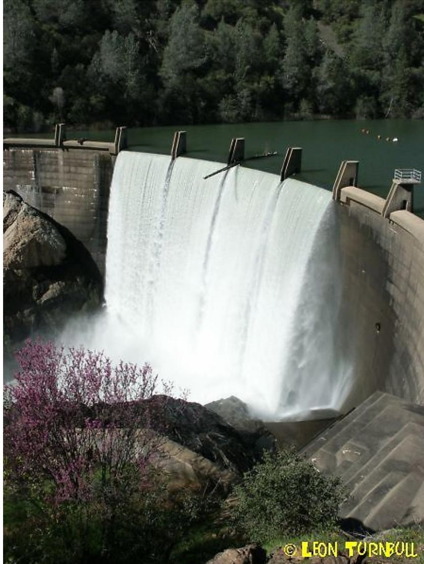
Figure B.7. Ogee weir at North Fork Debris Dam forming Lake Clementine. USGS gage 11427000 is on the bank of the lake approximately 50 feet upstream of the dam. Apparently, there are no low-flow outlets. (Photo used with permission from Leon Turnbull, see also [www.waterfallswest.com](http://www.waterfallswest.com))
