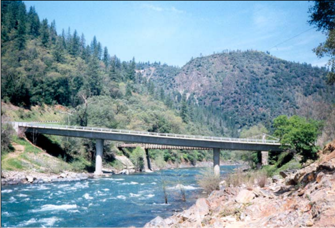
Figure 2. Colfax-Iowa Hill Bridges over North Fork American River
