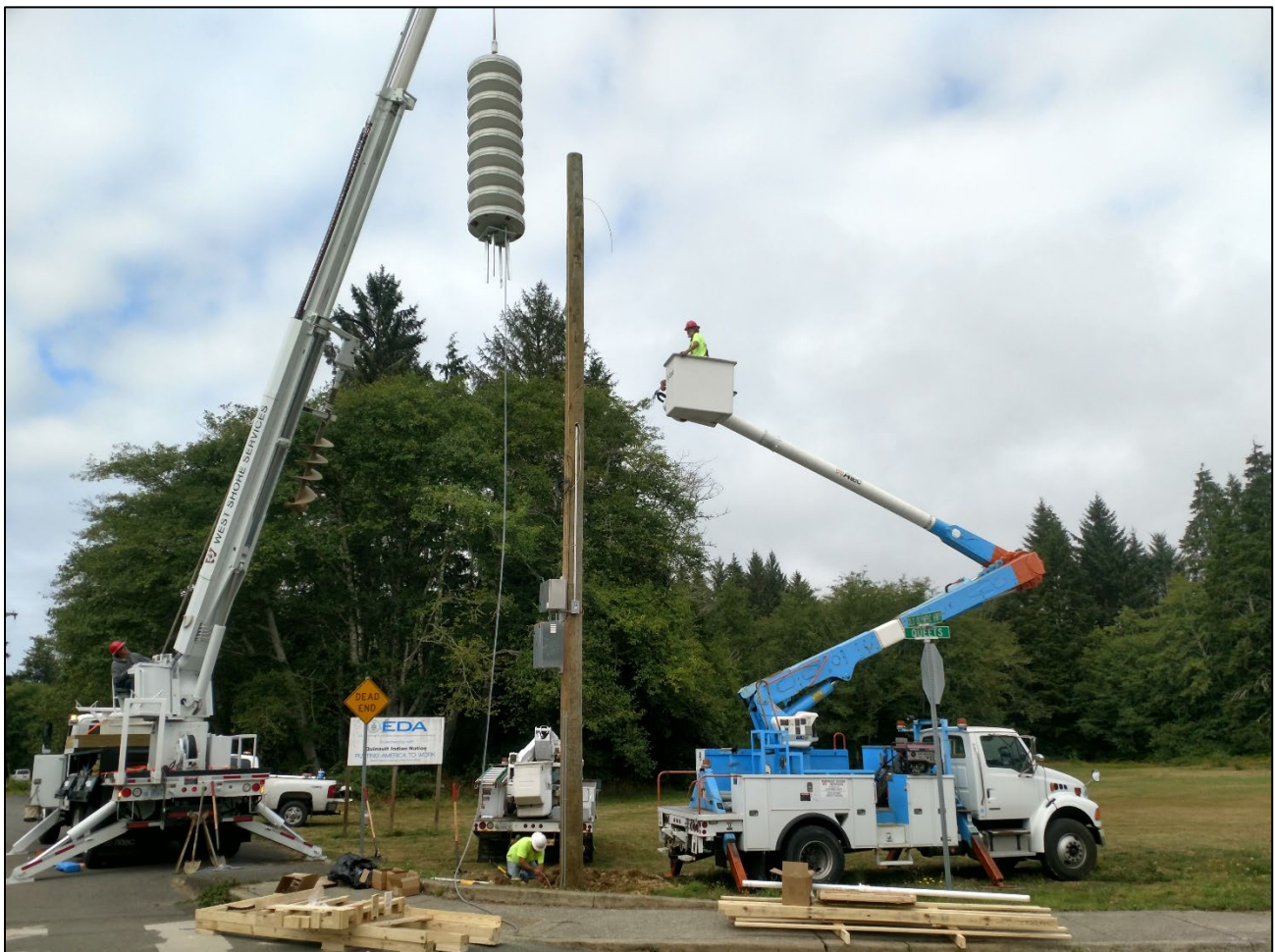
Sirens can alert people of an imminent tsunami, providing they have been trained to understand and respond to an alert. Here is a siren being installed along the Washington coast. (WA Emergency Management Division)
