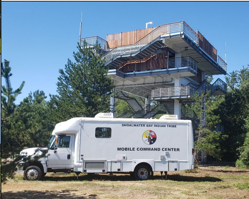
Vertical-evacuation structures provide places for people to escape tsunami waves if there is not enough time to reach natural high ground. Examples include a rooftop refuge at Ocosta Elementary School near Westport, WA (upper left), a rooftop refuge at the Hatfield Marine Science Center in Newport, Oregon (lower left), and the Auntie Lee Vertical Evacuation Structure in Tokeland, Washington (right).
