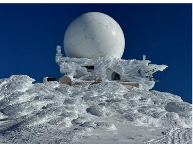
Here are some other fun facts about our radar: It is located at 7,532 feet, is the 2nd highest National Weather Service radar in the Contiguous United States, and it is set at a -0.2° elevation scan. With most NWS radars, the scanning begins with 0.5° elevation meaning the centerline of the radar beam antenna is angled 0.5° above the ground. Why in the world would we set our radar to a -0.2° elevation scan? With our radar at over 7,500 feet, we need to see what is happening below it!
