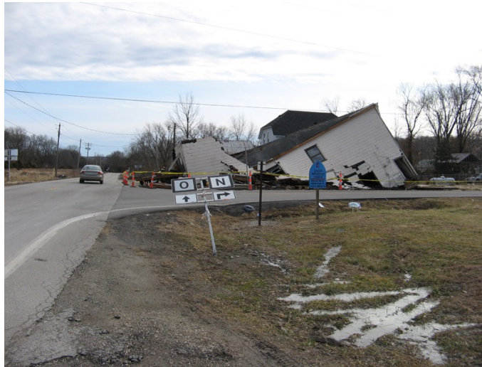
Above: EF2 tornado damage in Robertsville, MO (Franklin county)
