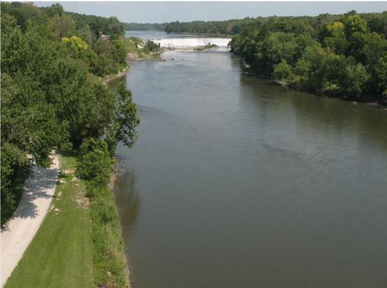
Fox River at Dayton Dam – Typical
