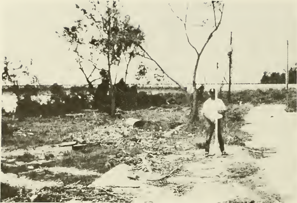
Photo 1. Surveying debris line at the east end of old Highway 90 fishing bridge, Biloxi, Miss.
