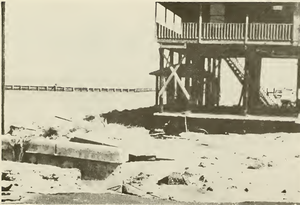
Photo 4. Foundation damage on the western half of Dauphin Island, bay side
