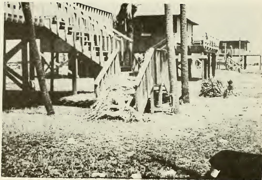
Photo 9. Debris line on house steps near Gulf Shores, Ala.
