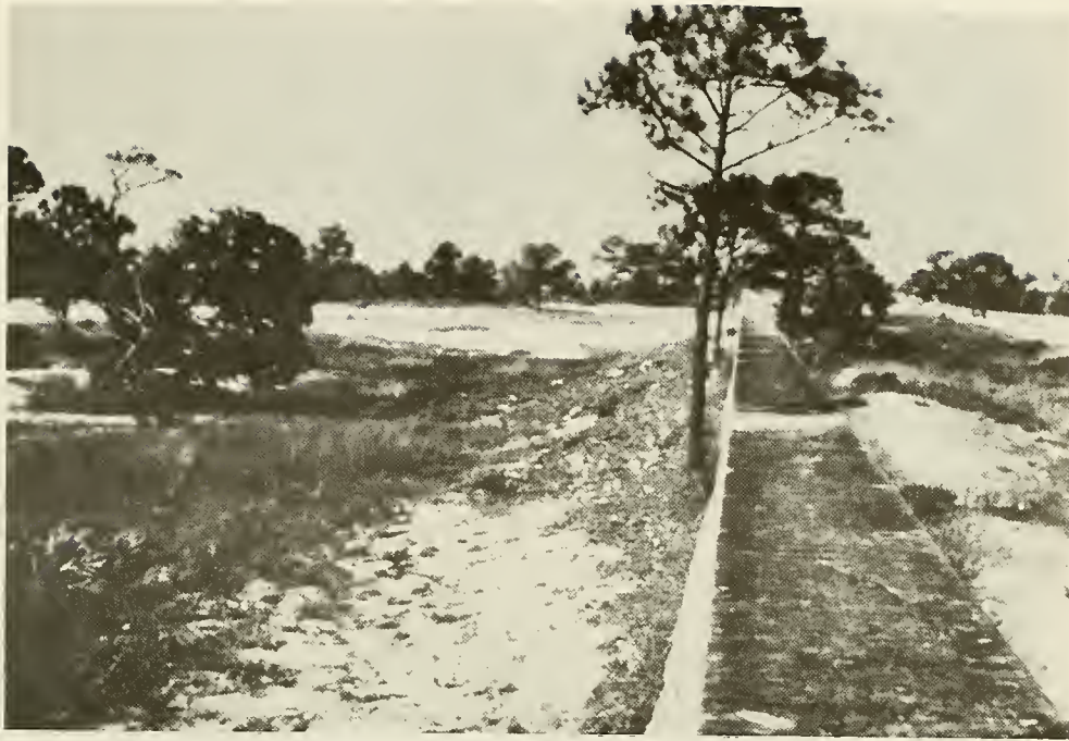
Photo 7. Debris line at the foot of the seawall, Ft. Morgan State Park, Ala., looking west
