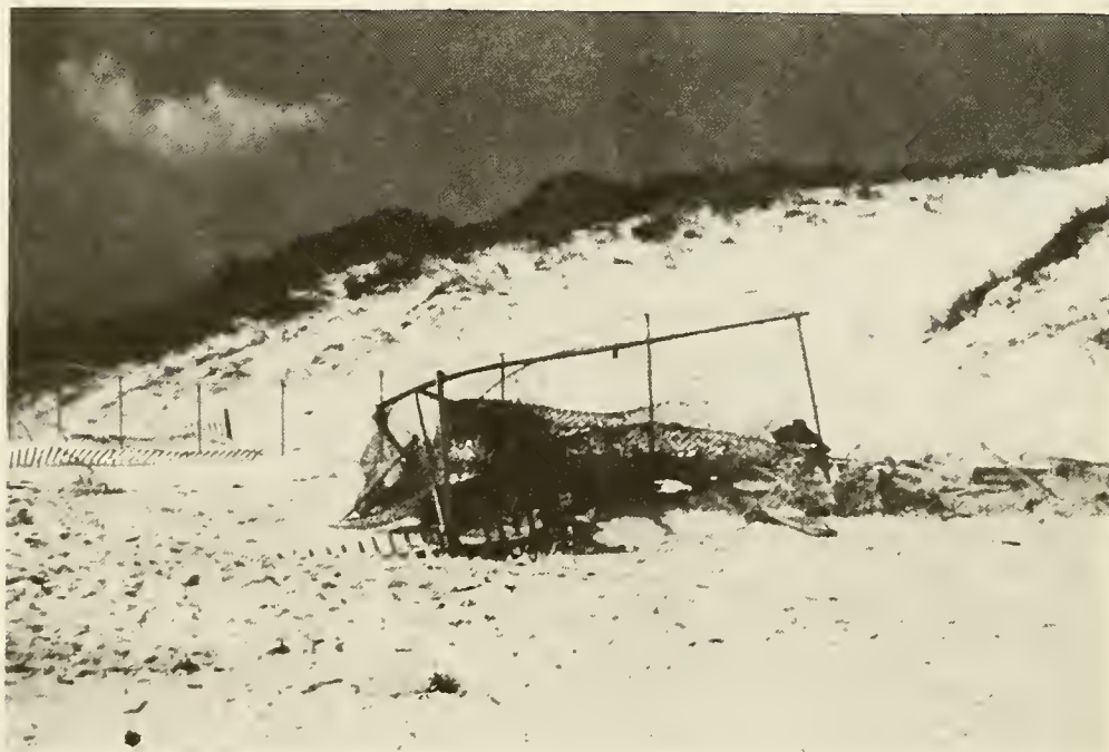
Photo 10. Damage to chain link fence in front of dune line at Pensacola Beach, Fla.
