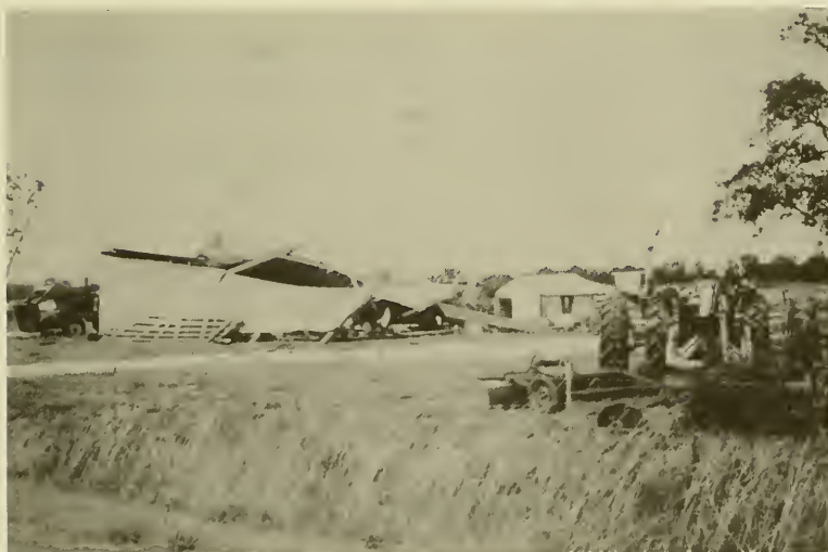
Photo 6. Collapsed farm equipment shed near Intracoastal City, La.
