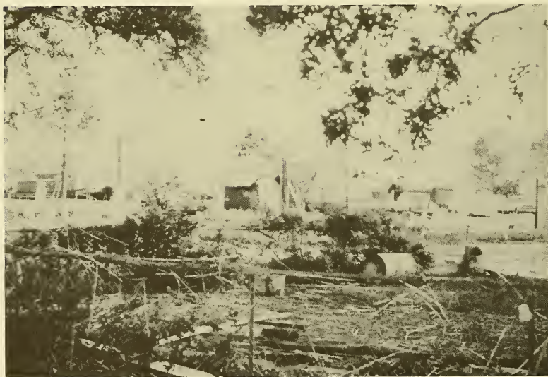
Photo 4. Debris line on fence, Intracoastal City, La.
