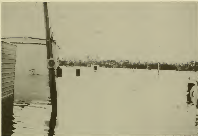
Photo 5. Residual flooding of the air logistics base near Intracoastal City, La.
