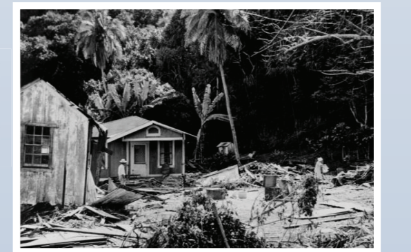
Left: Tsunami damage near Kalihiwai Bay, Kaua'i (1946). Image credit: O Magoon
