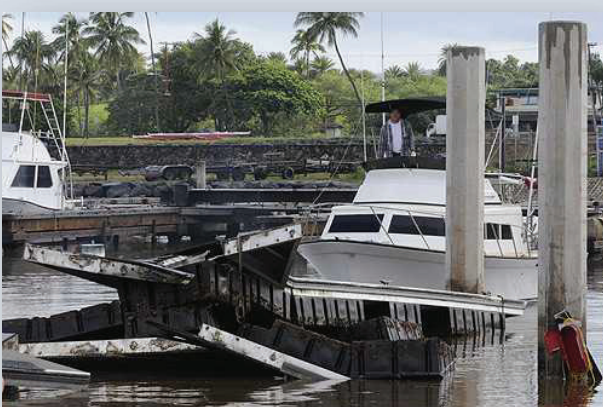
Images show damage in the Haleiwa Harbor on Oahu from the 2011 Tohoku, Japan tsunami. 2 m runup height. Image credit: Mader Consulting Co.
