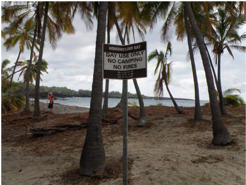
Figure B13d. Signage bent by force of tsunami at Honomalino Bay, Ka'u.
