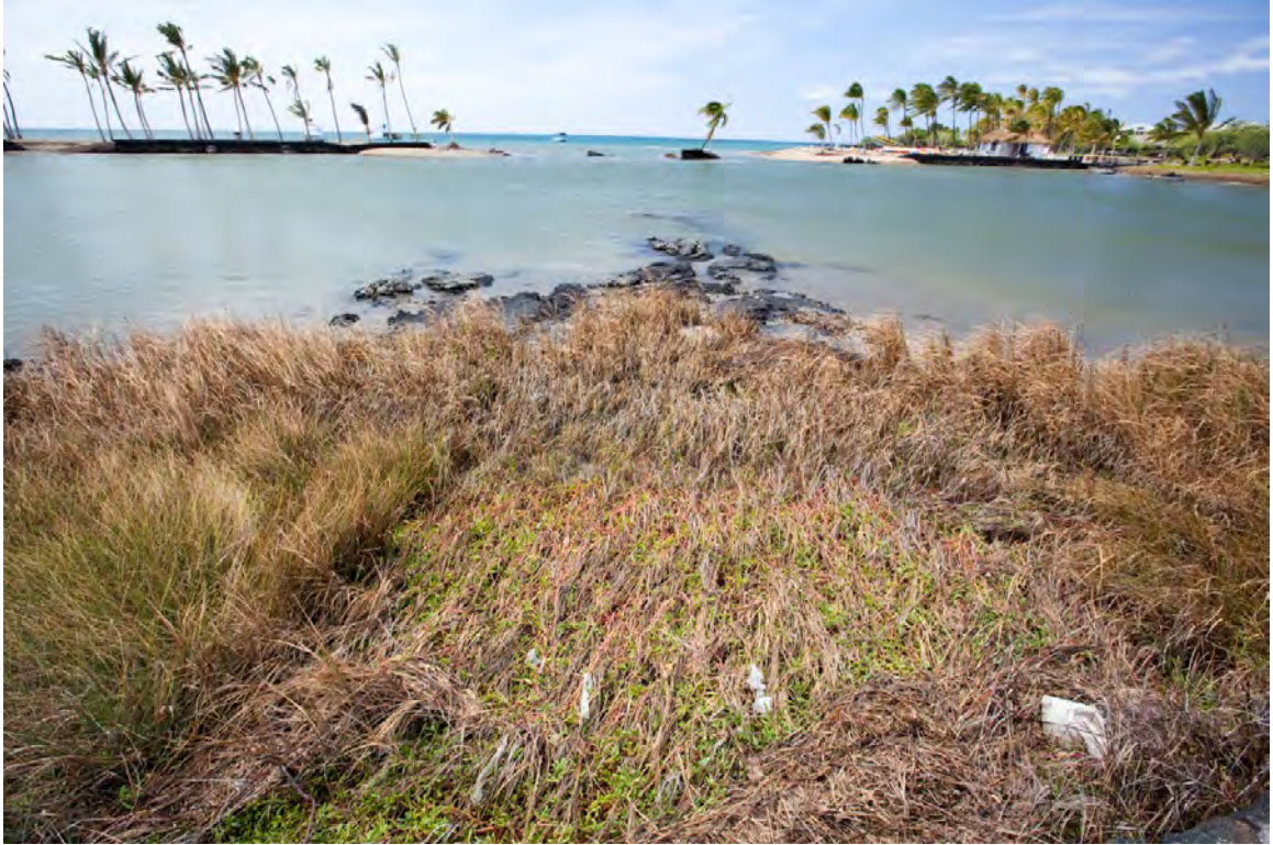
Figure B25c. Fishpond breached by tsunami. View northwestward.
