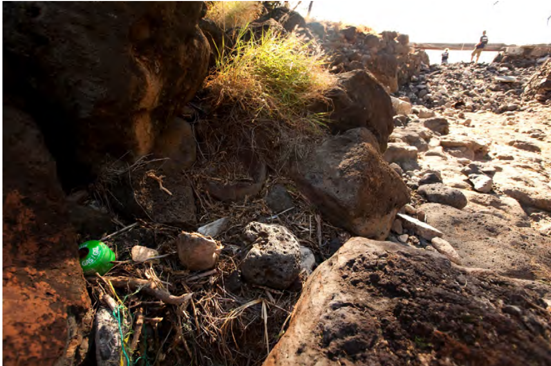
Figure B27b. Debris swept inland up drainage ditch near old wharf at Mahukona Beach Park.
