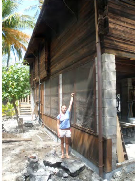
Figure B24b. Private home with breakaway walls. Structure sustained minimal damage.
