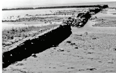
E-53, Fishpond walls at Pukoo, Molokai, broken by Tsunami.
