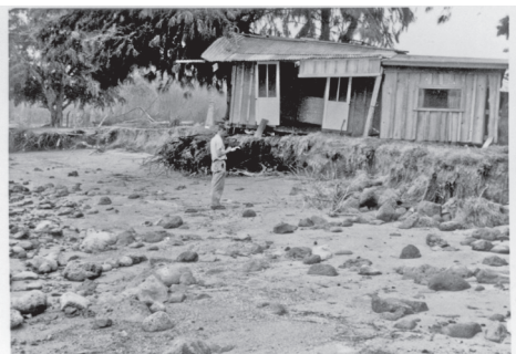
E-51, Damage to house, and scarp formation at head of beach, at Kainalu, Molokai.
