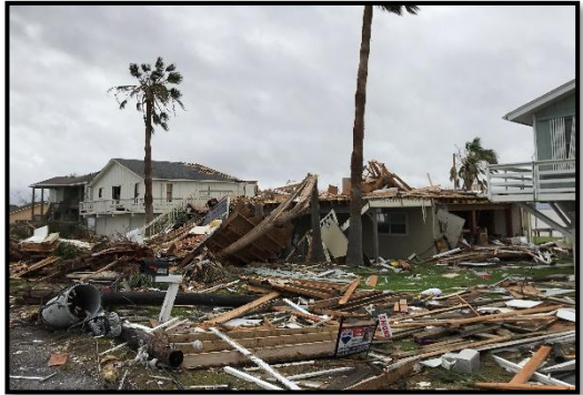
Above: Damage to the community of Copano Village in Aransas County, TX in the wake of Hurricane Harvey in 2017.
