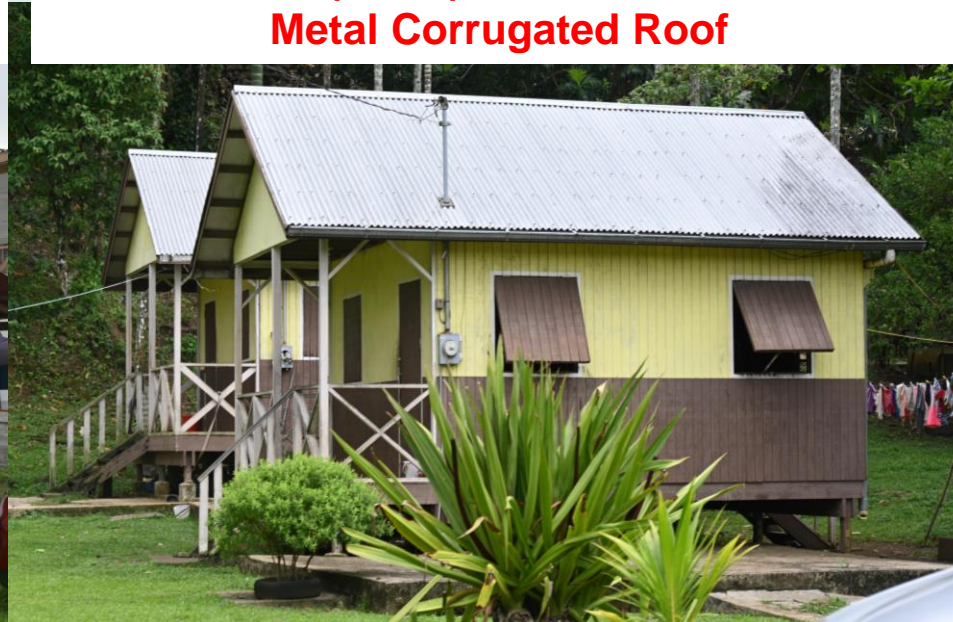
Wood Walls (studs) & Wood Framed Roof - Metal Corrugated Roof
