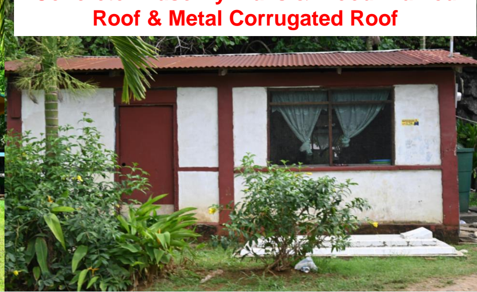
Wood Walls (T1-11), Wood Framed Roof & Metal Corrugated Roof
