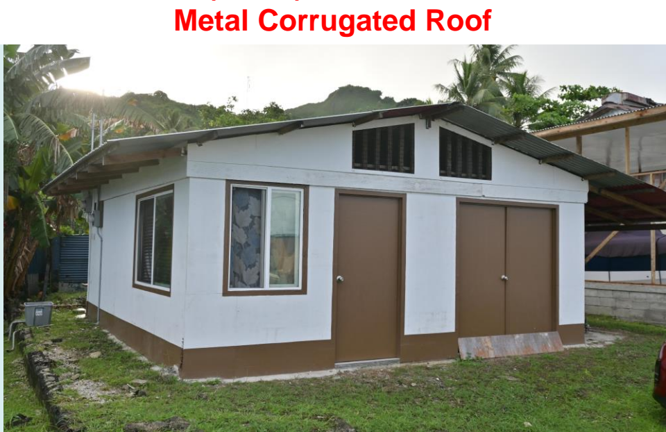
Wood Walls (T1-11), Wood Framed Roof & Metal Corrugated Roof
