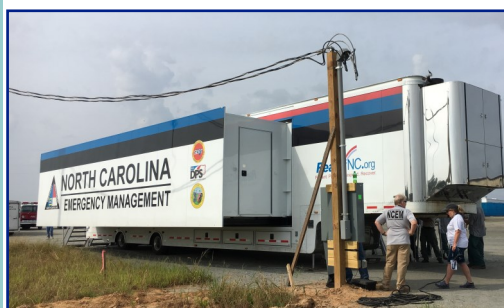
This portable facility is owned by North Carolina Emergency Management. It served as the Emergency Operations Center for the WEG.
