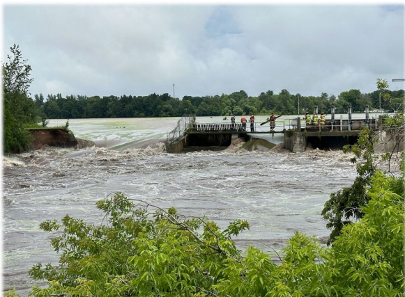
Manawa Dam failure
