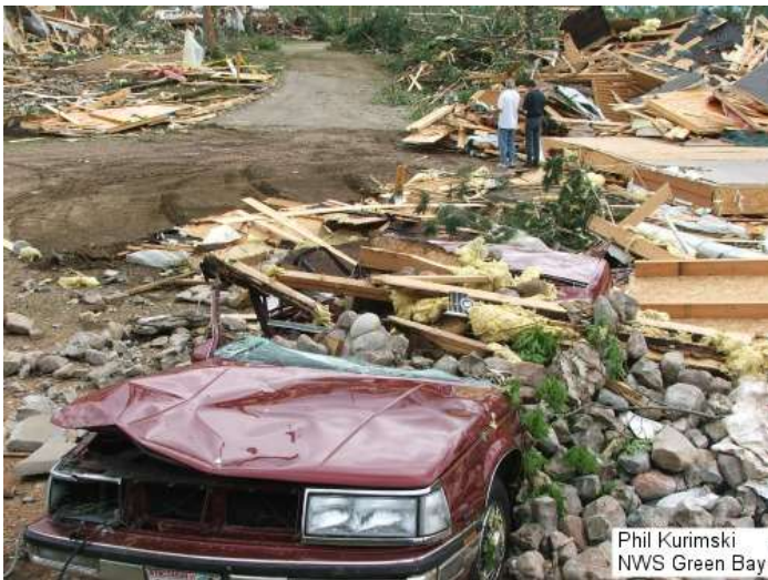
Picture on the left: More damage at the Bear Paw Resort.
