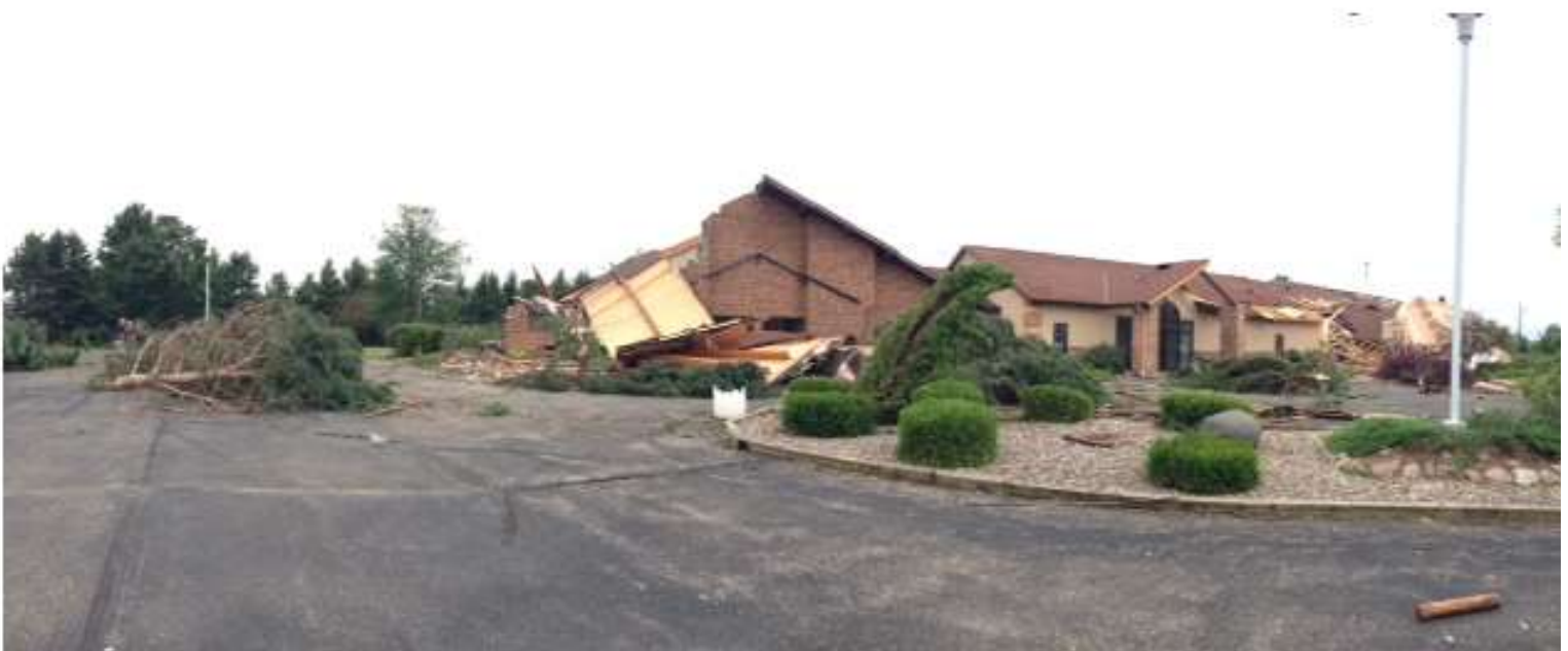
Figure 1: Church (southeast New London) damaged by a tornado. Peak winds were estimated at 115 to 120 mph.
