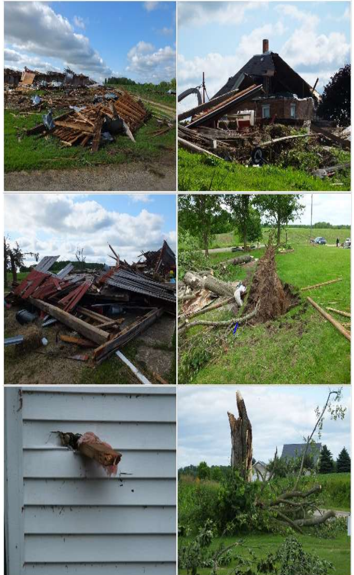
Here are some damage photos from the Marion tornado:
