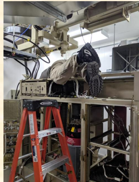
Image 2: Installing the new wiring harness in the radar transmitter. Credit: NWS
