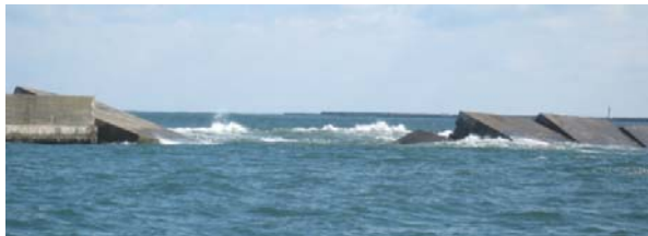
Photo 8 Caisson sliding at Hattaro Breakwater in Hachinohe Photo 9 Seawall at Ryoishi in Kamaishi
