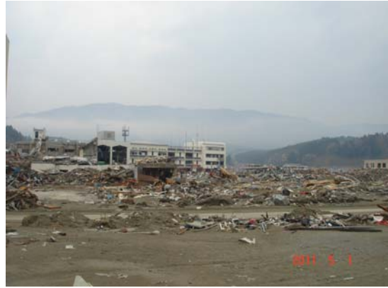
Photo1(b) Flattened wooden houses and remaining concrete buildings(Rikuzen-Kakada)
