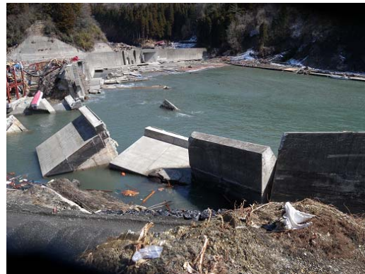
Photo 8 Caisson sliding at Hattaro Breakwater in Hachinohe Photo 9 Seawall at Ryoishi in Kamaishi
