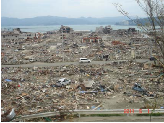
Photo 1(a) Flattened wooden houses and remaining concrete buildings(Minami-Sanriku)
