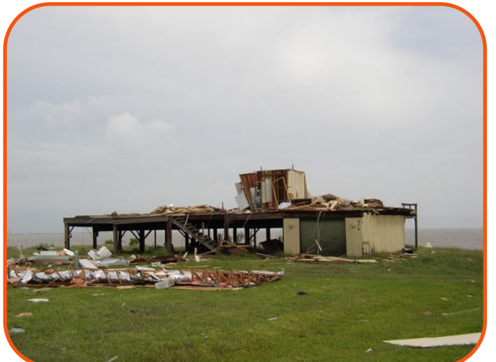
House destroyed in Alamo Beach
