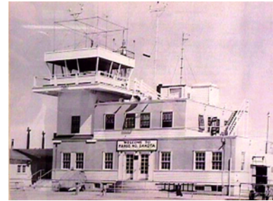
d) Airport Administration Building, Fargo, ND
