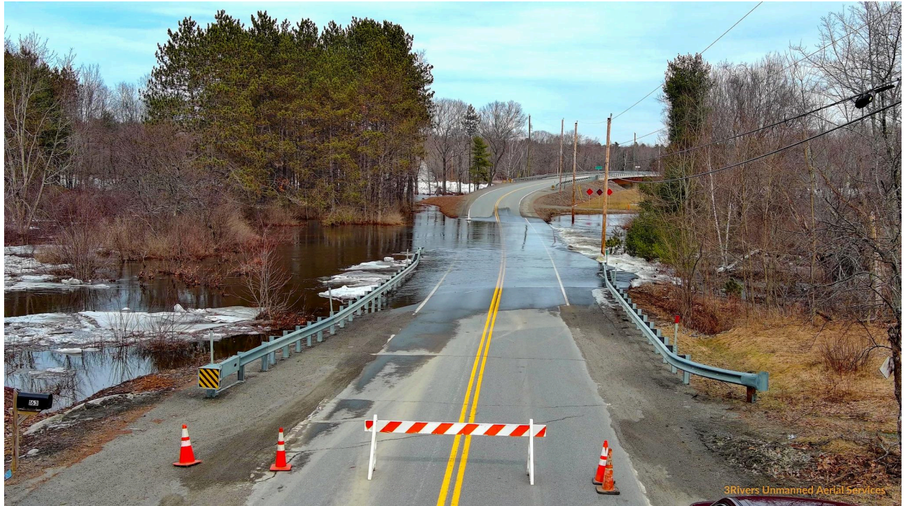
Pleasant River @ Milo Pleasant St. Bridge on March 18, 2025 Courtesy: Piscataquis County Emergency Management
