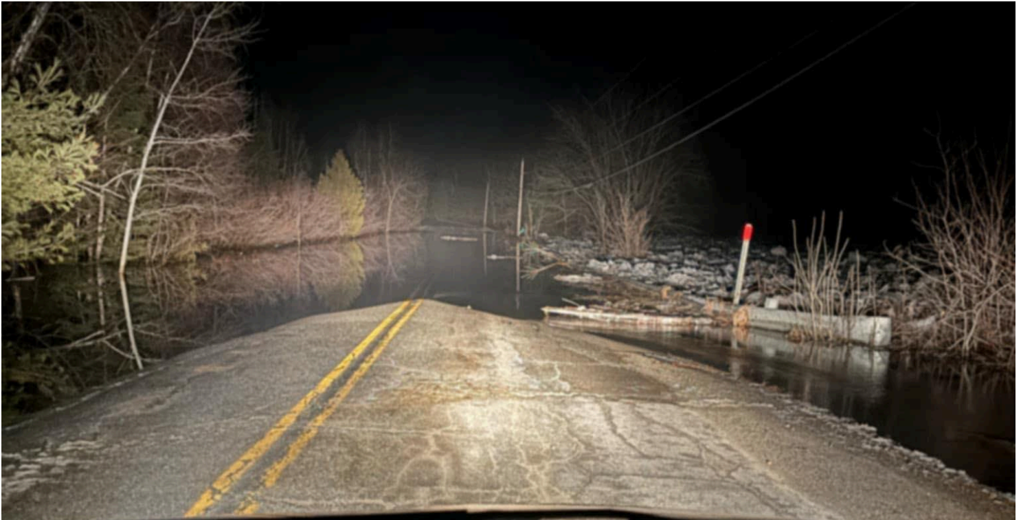
Reed Plantation on March 19, 2025 Courtesy: Aroostook County Flood Watch
