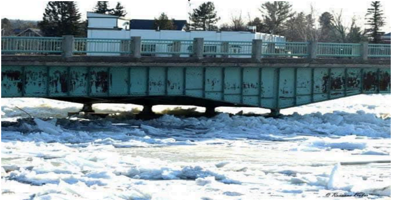
December 16, 2024 - Aroostook River - Fort Fairfield Ice Jam - Route 1A Bridge Photo Courtesy: Roxanne Bubar
