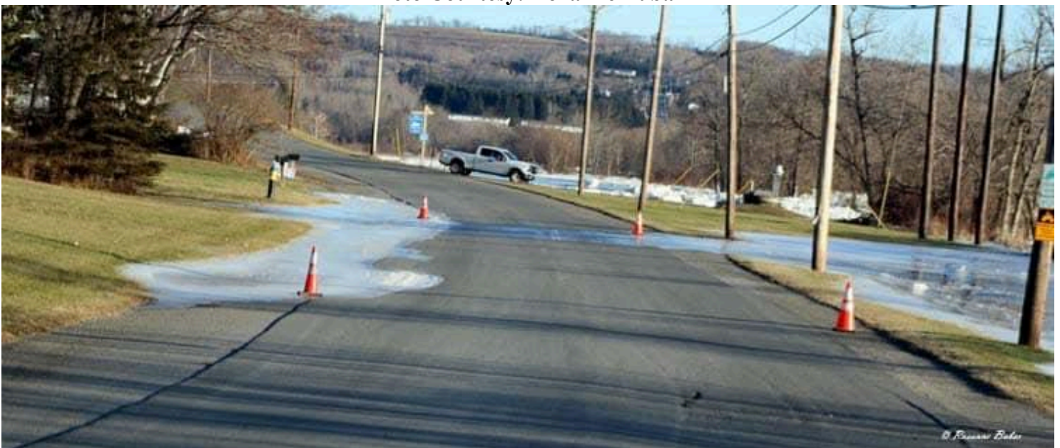
December 16, 2024 - Aroostook River - Fort Fairfield Ice Jam - Russell Rd Minor Flooding Photo Courtesy: Roxanne Bubar
