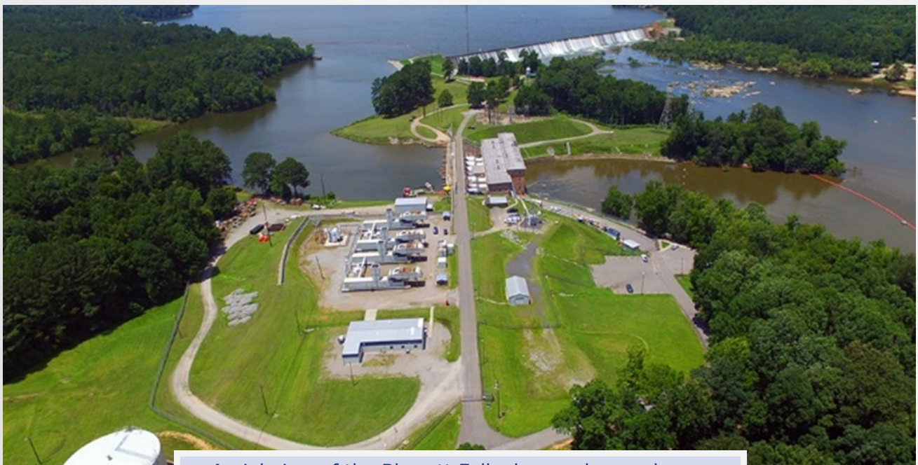
Aerial view of the Blewett Falls dam and powerhouse
