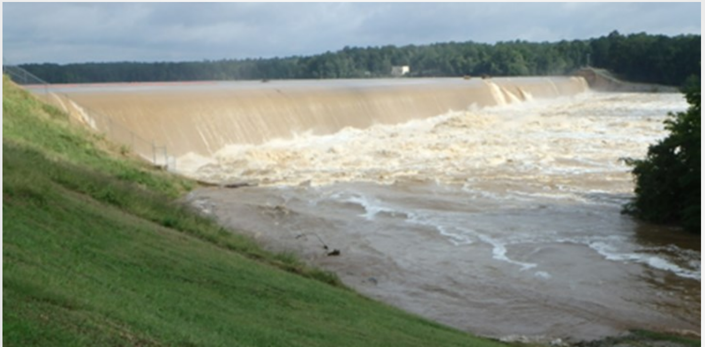
Water flowing over the Blewett Falls Dam during the flooding produced by Hurricane Florence
