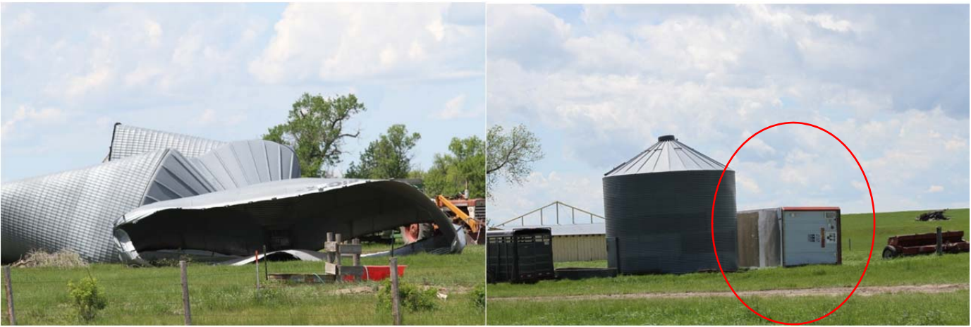
Figure 3: Grain Bin Damage and Semi-Trailer tipped on its side
