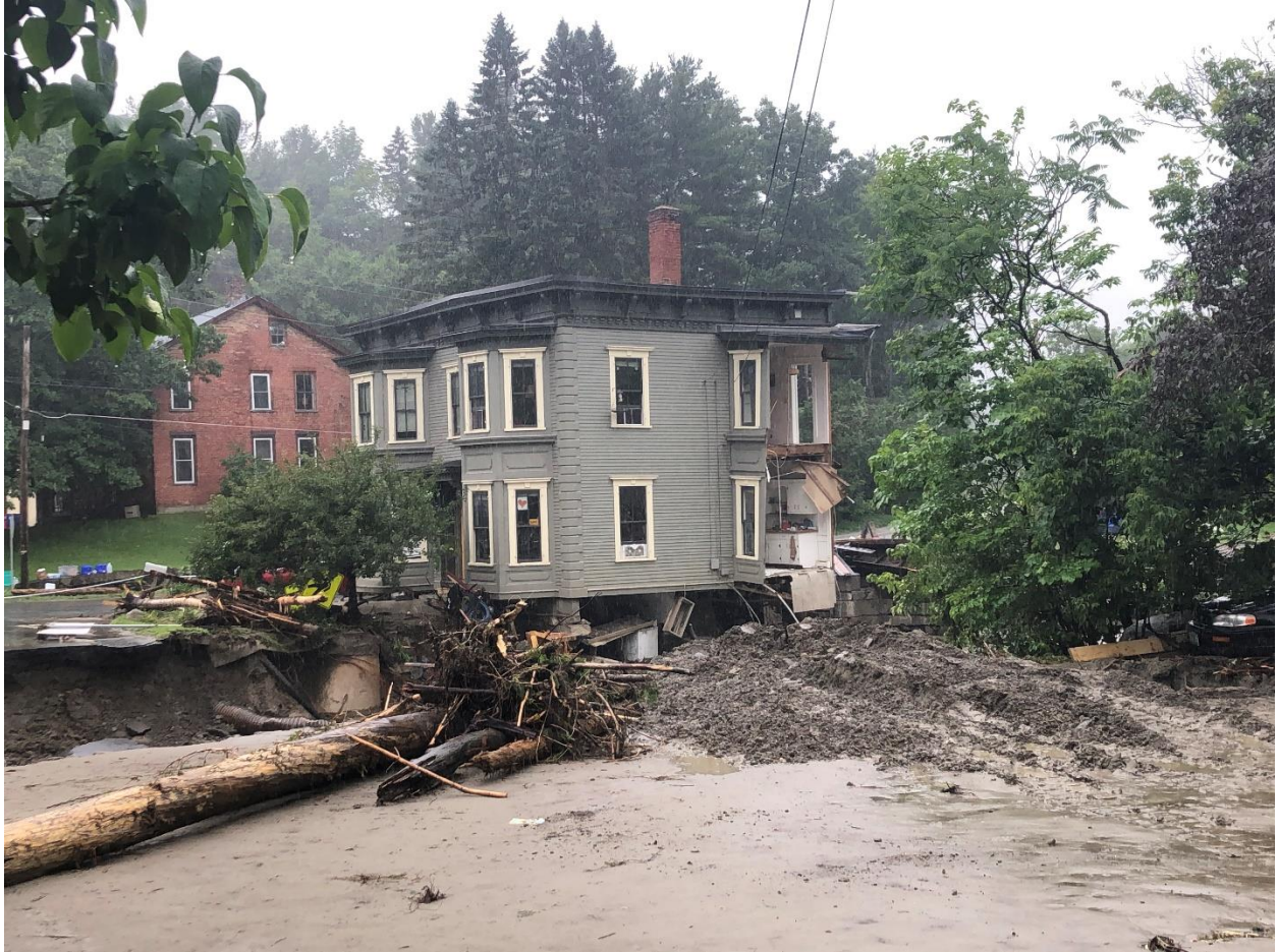
Figure 5: Significant flash flooding late on July 10 led to catastrophic damage in the Plainfield, VT area, including this apartment building that was almost completely washed away by the Great Brook.
