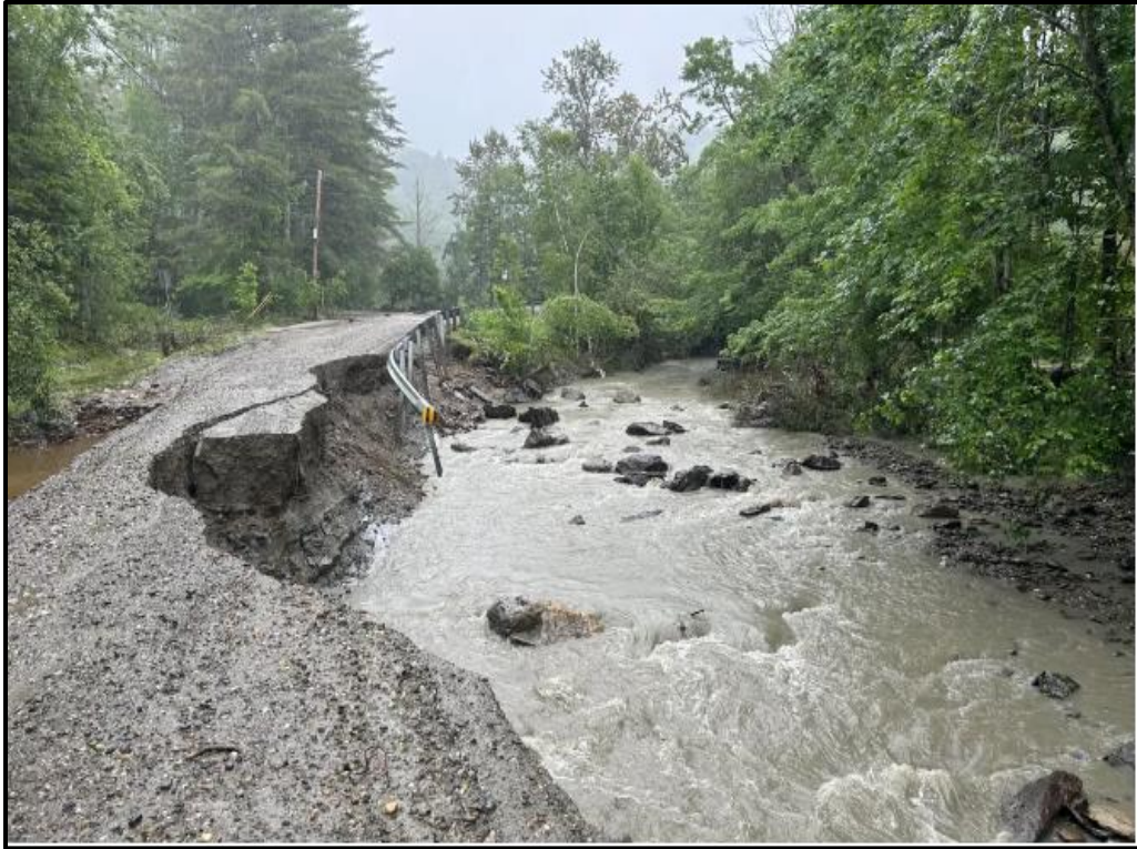
Figure 5: Significant flash flooding on the evening of June 23, 2024 led to numerous road washouts in the Stowe, VT area, including Moss Glen Falls Road, shown here (picture courtesy Stowe, VT Public Works).
