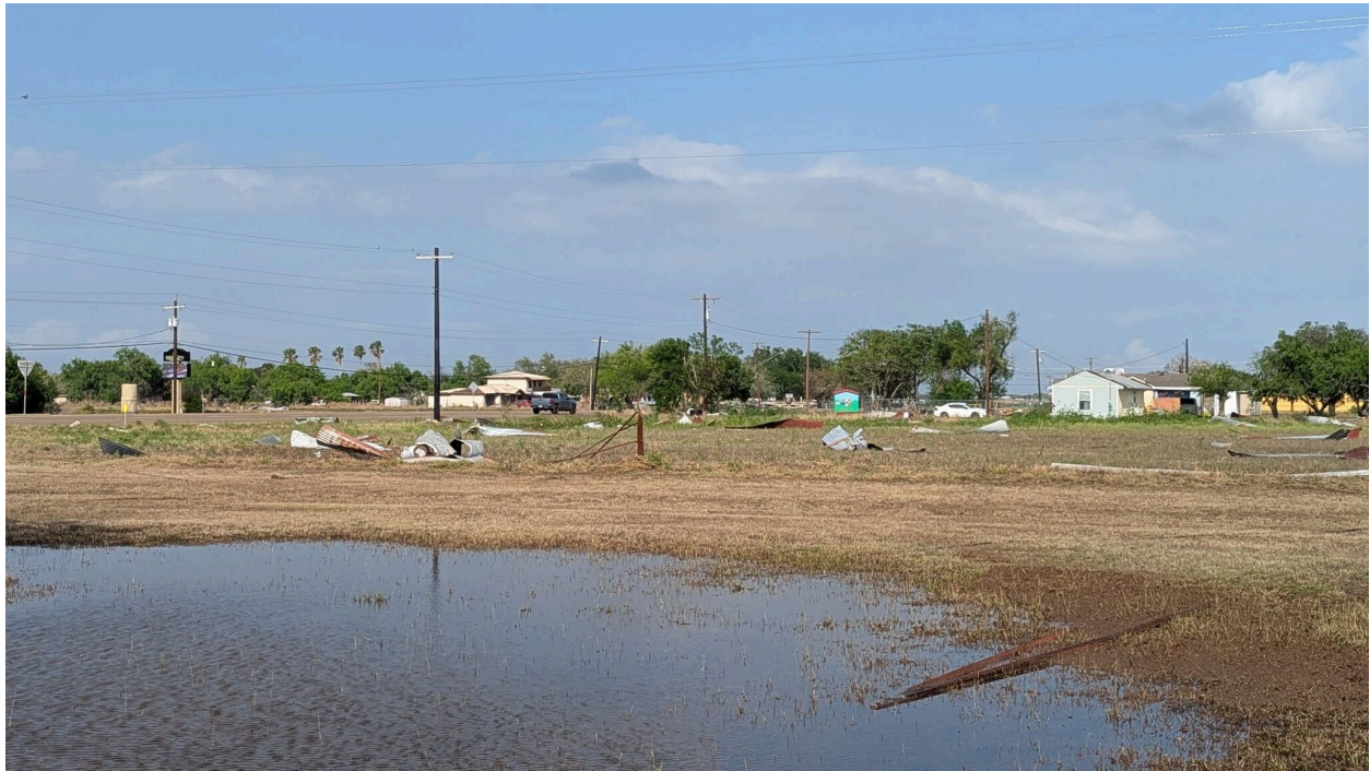
Above: Debris from the crop dusting business building that received a direct hit from the EF-0 tornado in Edcouch, TX (NWS Storm Damage Survey Team)
