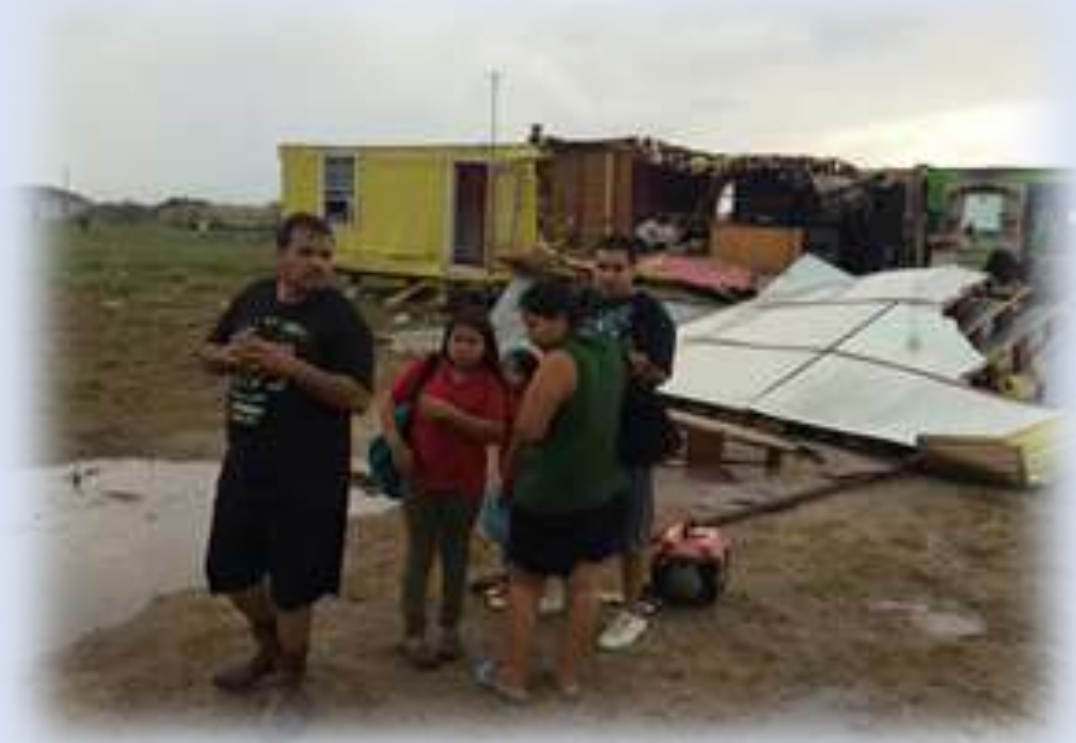
Photo of destroyed stick-built residence in a colonia near Alton, TX, following a severe thunderstorm in 2015.
