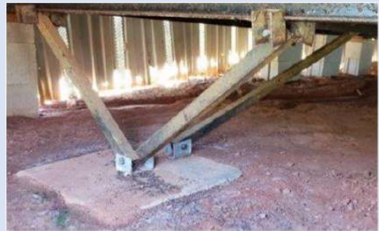
Figure 2: Example of pan anchorage for a pier-block foundation residential construction. From Analysis of Manufactured Home Vulnerability in Extreme Winds , Davis, B. M., 2020.
