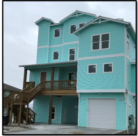
Above: This well built home in the community of Copano Village in Aransas County, TX survived Hurricane Harvey in 2017.
