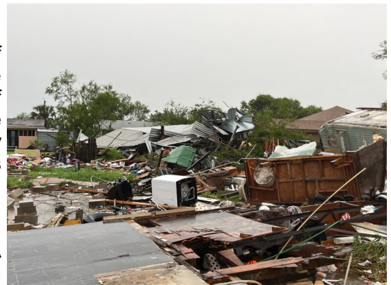
Above: Demolished substandard buildings in Laguna Heights, May 13, 2023
