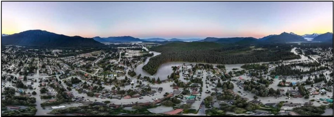
Multiple areas experienced major flooding, affecting approximately 290 homes, some of which were inundated with 4 to 6 feet of water. (Photo Credit - Alaska Senator Lisa Murkowski, via Facebook )
