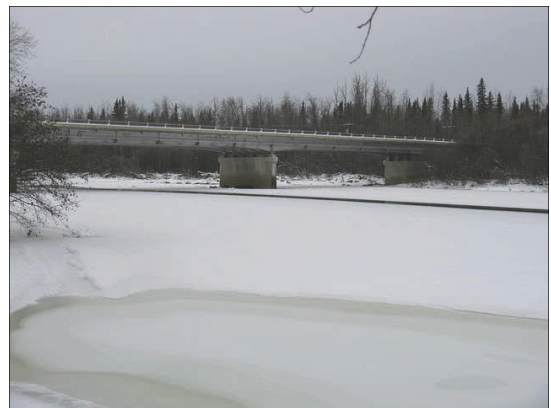
Freezeup at the Salcha River Bridge
