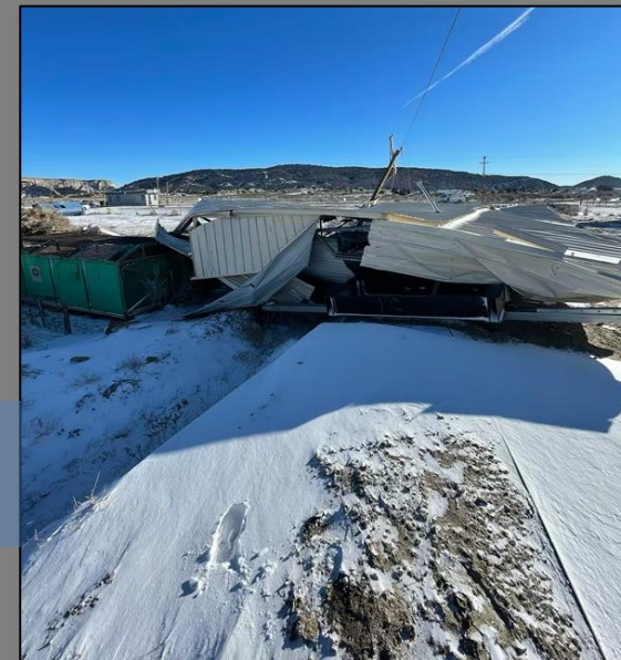
COVID Test Site Wind Damage | Dec. 15, 2021 Courtesy of Frank Kozeliski
