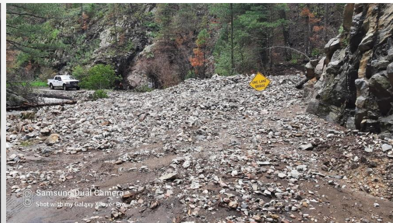
July 29 Gavilan Creek flood Photo courtesy Ira Pearson
