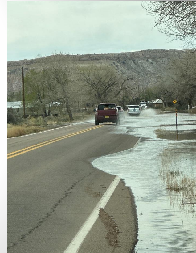
Photo courtesy NMSP Jemez River Flooding
