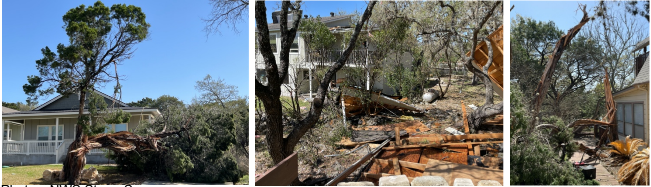
Photos: NWS Storm Survey
