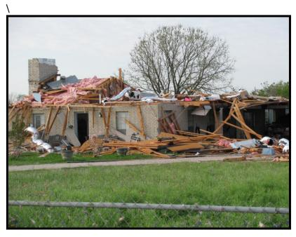
Figure 8. A home severely damaged By the EF2 Tornado in southwestern Bexar County, TX, on March 19, 2012.
