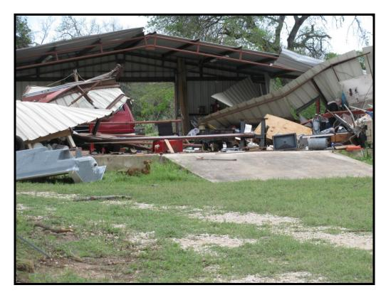
Figure 5. A steel frame shed severely damaged by the EF1 Tornado near Natalia, TX, on March 19, 2012.
